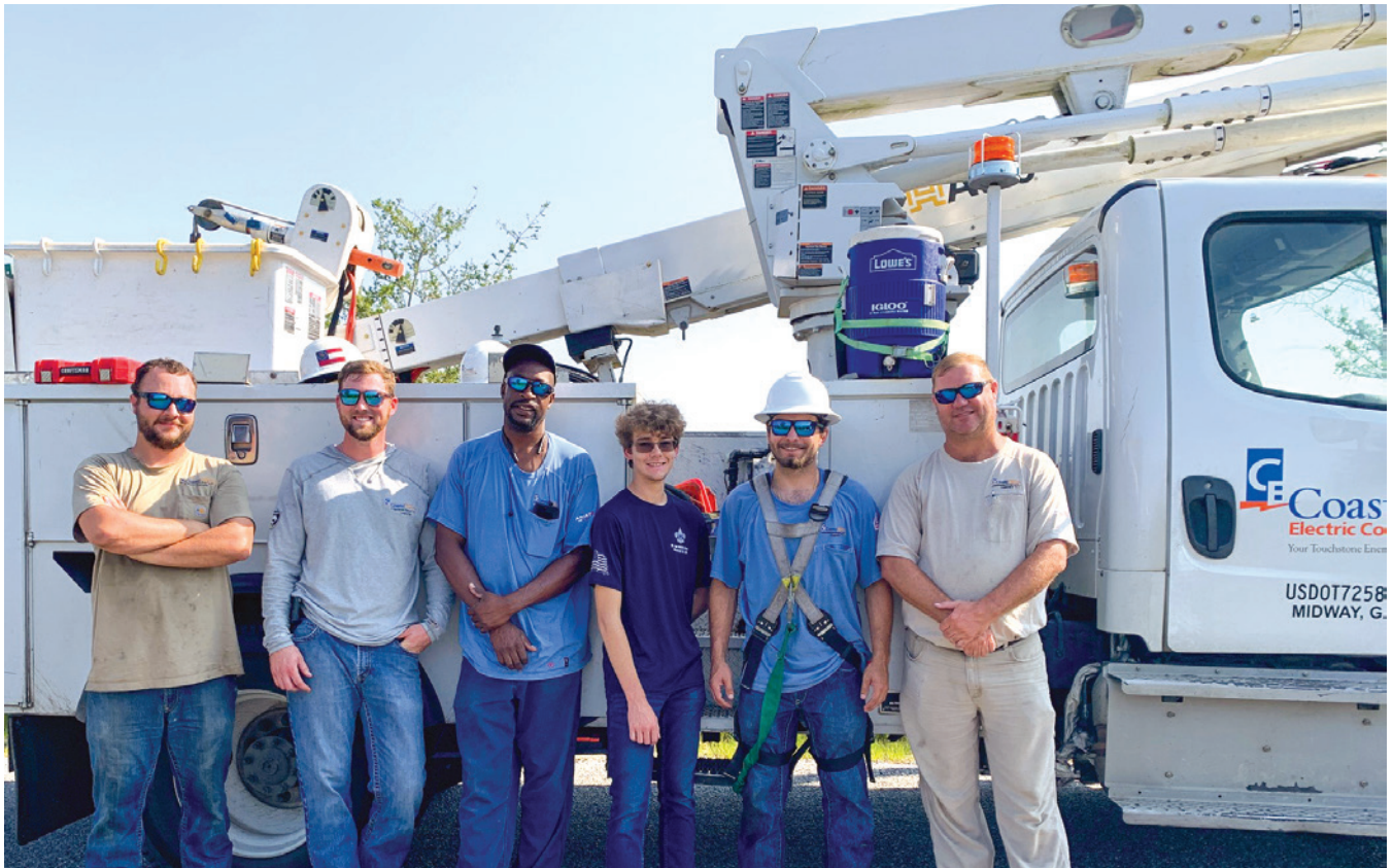
What a crew! Coastal Electric Linemen Josh Cowart, Slade Walker, Eric Wells, Hunter Hawkins and Clint Durrence finish installing bat boxes, built by Boy Scout Randall Singhas (third from right).
